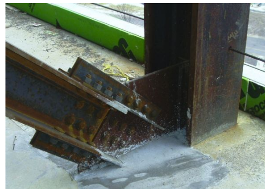
Figure 10 - Diagonal Brace Connection at Column Photo Courtesy of Jim Boje, PE (Wendel)
